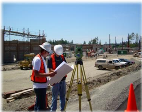
Figure 7.1 Surveying is being carried out on the construction site
